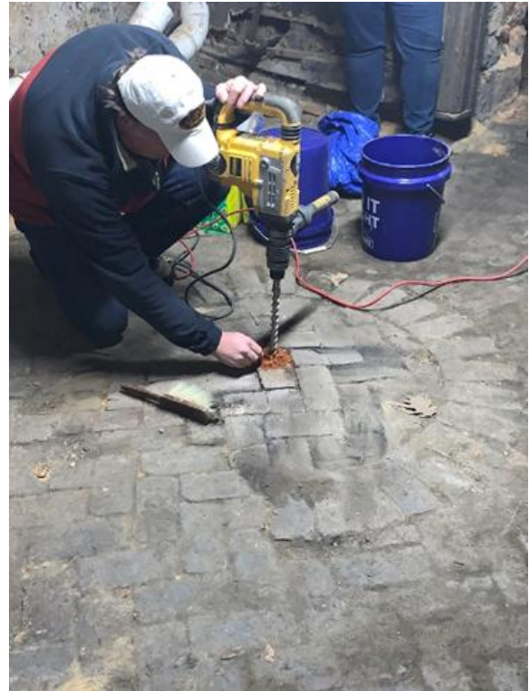
Holes were drilled through the brick cover of the enclosed well
